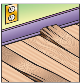
▲ loose floorboards
